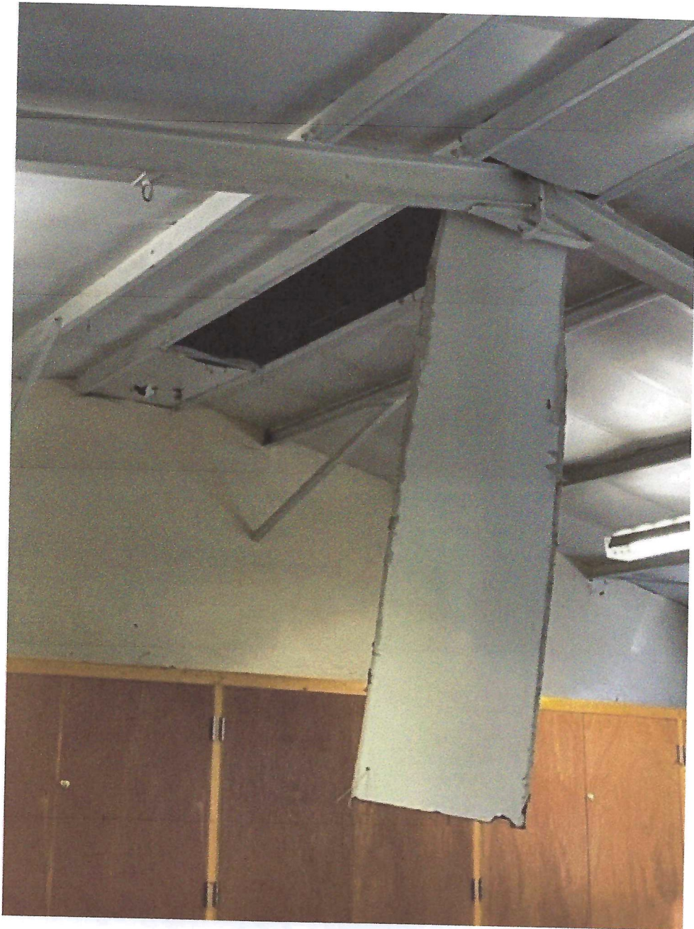
Photos from Building Inspection 18/11/2022
