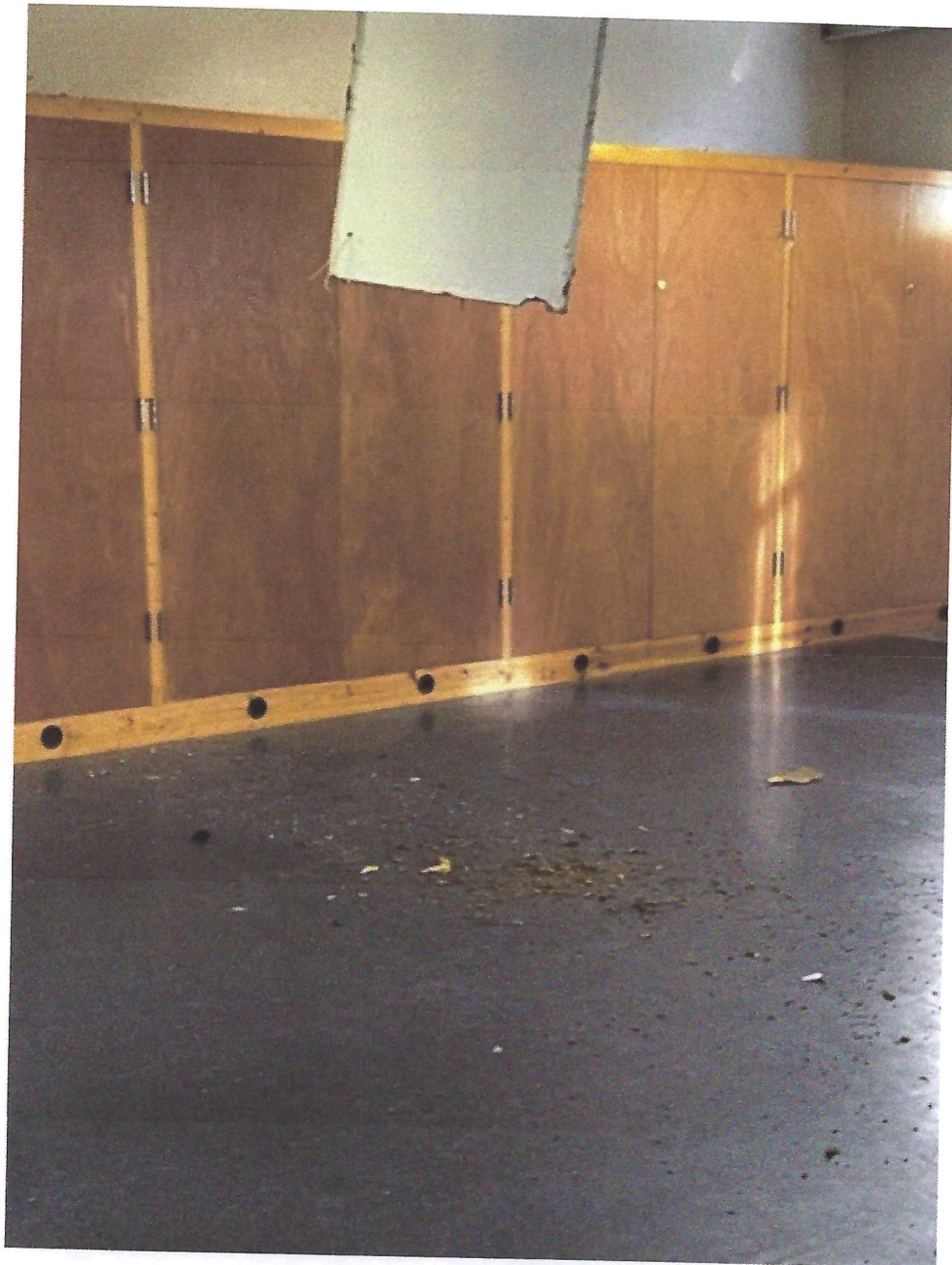
Photos from Building Inspection 18/11/2022
