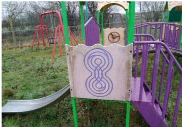
**Finding:** The height of the barrier(s) is insufficient and fails to meet the requirements of BS EN 1176 Part 1
