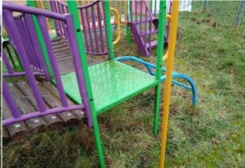
**Finding:** The free space between the fireman's pole and the **Action:** Monitor - No remedial work recommended platform is less than the minimum recommended dimension of 350mm in BS EN 1176 Part 1; this is however an intended design feature by the manufacturer to assist younger users in accessing the pole and is a very low risk finding - no remedial action is recommended
