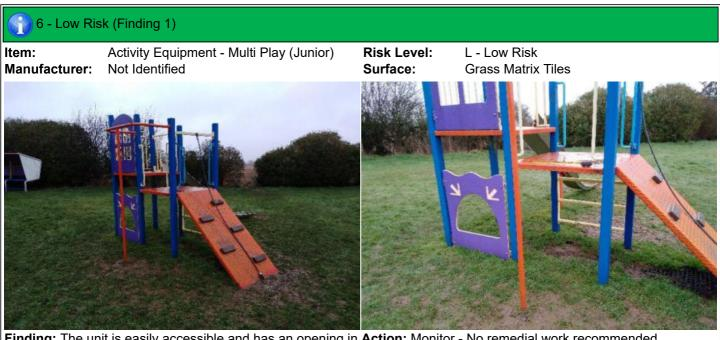
**Finding:** The unit is easily accessible and has an opening in **Action:** Monitor - No remedial work recommended the barrier to steep play elements in excess of 500mm in contravention of BS EN 1176 Part 1
