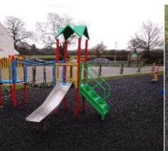
**Finding:** The height of the slide runout is in excess of 200mm and fails the requirements of BS EN 1176 Part 3
