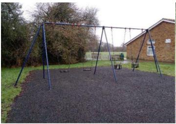
Finding: The seats are too close to the frame as defined in Action: Monitor - No remedial work recommended BS EN 1176 Part 2; this is a low risk failure and no remedial action is required
