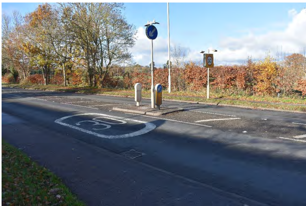
Traffic island in Hatfield Road.
